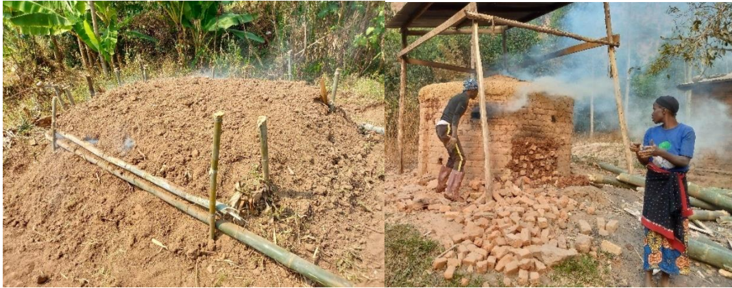
Fig 7. Carbonization and aeration control: earth mound kiln (left), masonry kiln in bricks and clay (right)
